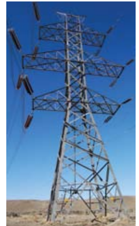
Vertical dead end, 500/230 kV, double circuit
