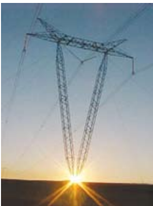
Horizontal guyed V, 500 kV
