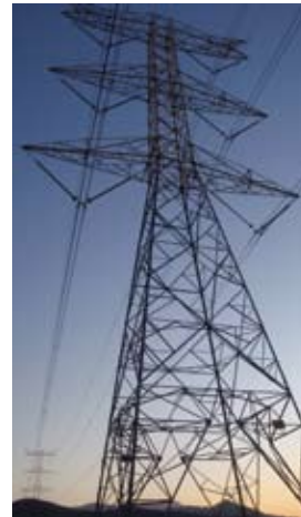
Vertical, 400 kV, double circuit
