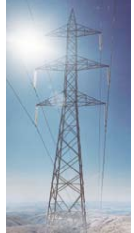
Vertical, 230 kV, double circuit
